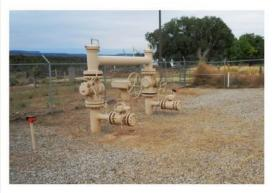
Mainline valves are an integral component of natural gas pipeline transmission systems. They function as gateways that, when open, allow the gas to flow freely or, when closed, stop the flow of gas or isolate a segment of the pipeline. They may be utilized during emergency
