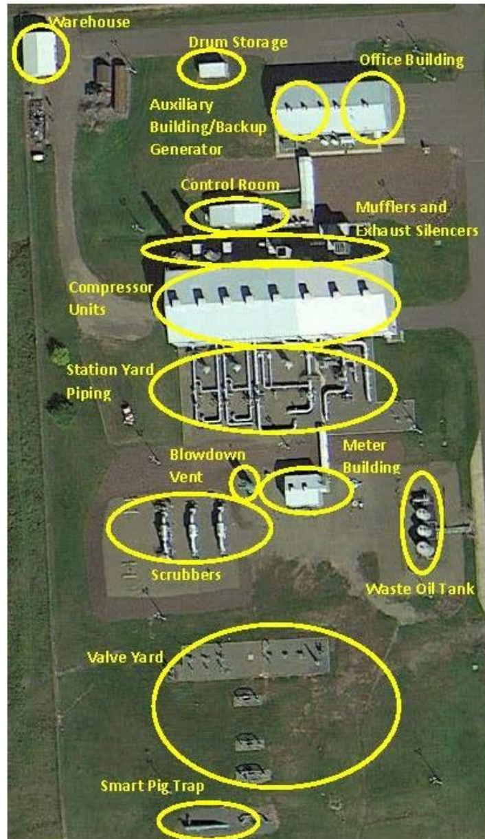
Figure 2-1. Typical Compressor Station
