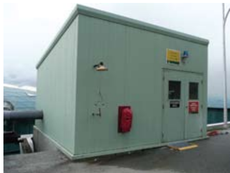
◀ Vapour Recovery Equipment Building
