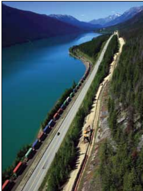
Anchor Loop construction through Mount Robson Provincial Park
