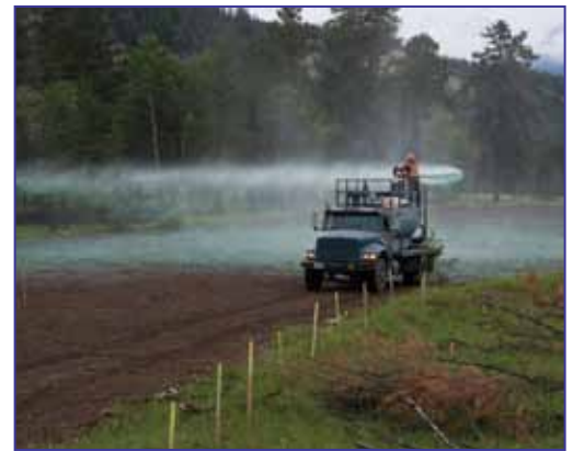
Hydroseeding on right-of-way
