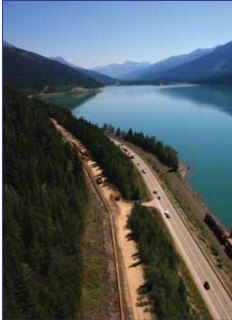
Anchor Loop construction
