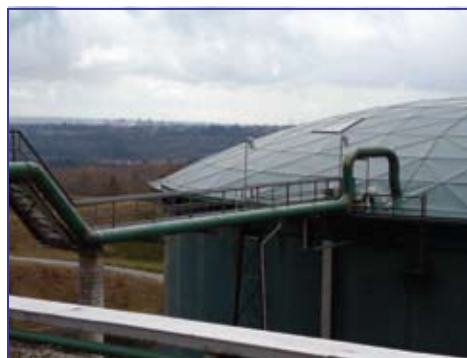
A domed roof tank at the Burnaby Terminal
