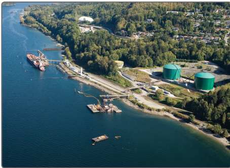
Westridge Marine Terminal
